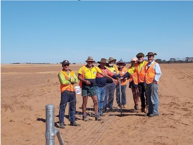
Blaze Aid Fencing after Fire
